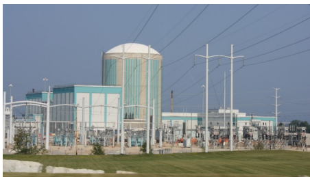
Kewaunee nuclear power plant, 2009
